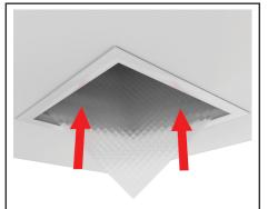
The diffuser can be installed by *gently* angling it and inserting up into the shaft.
