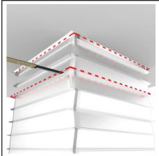
Using sharp knife and pliers/tinsnips, cut off excess flexi shaft 2 ribs below ceiling level.
