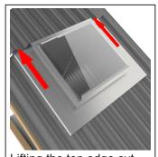
Lifting the top edge cut, slide the soaker tray up and under the cut. Rest the soaker tray on the roof sheeting. Secure the assembly into position by driving tech-screws through soaker tray into battens.
