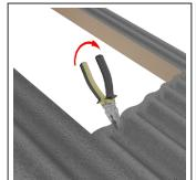
Weather up the corrugations on the low side of the cutout by folding the low spots with pliers.
