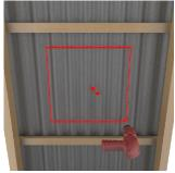
When satisfied with location, drill a hole in a bottom corner of throat position. Drill two holes above it to indicate direction of skylight.
