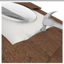
Using a hammer or rubber mallet, gently form the edges of the tray to match the roof profile.
